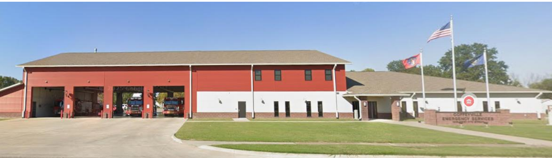
Photo: Google Maps, Photo captured, October 2025 Retrieved February 22, 2026
